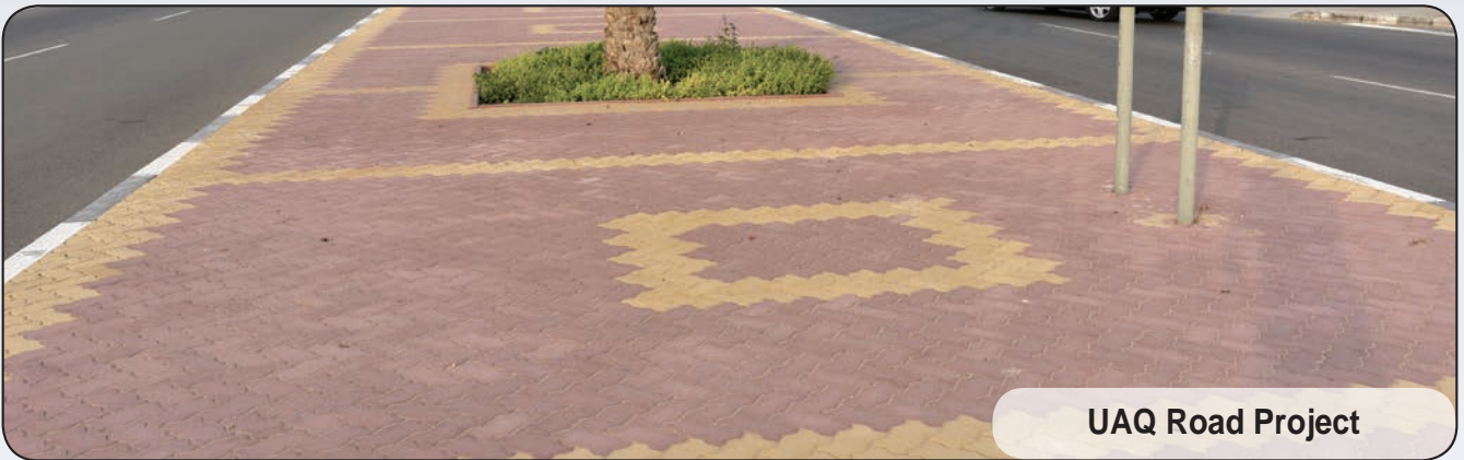
UAQ Road Project
